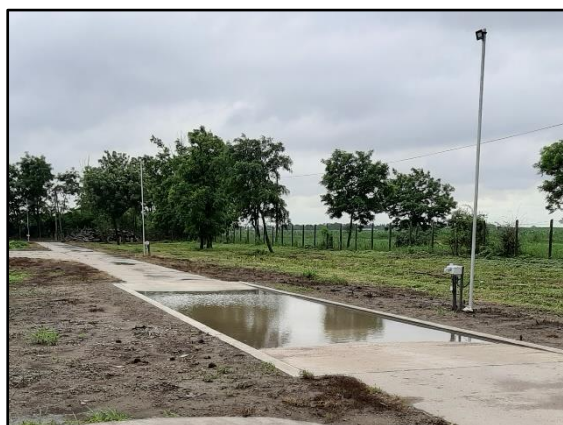
Water pit for incoming vehicles
