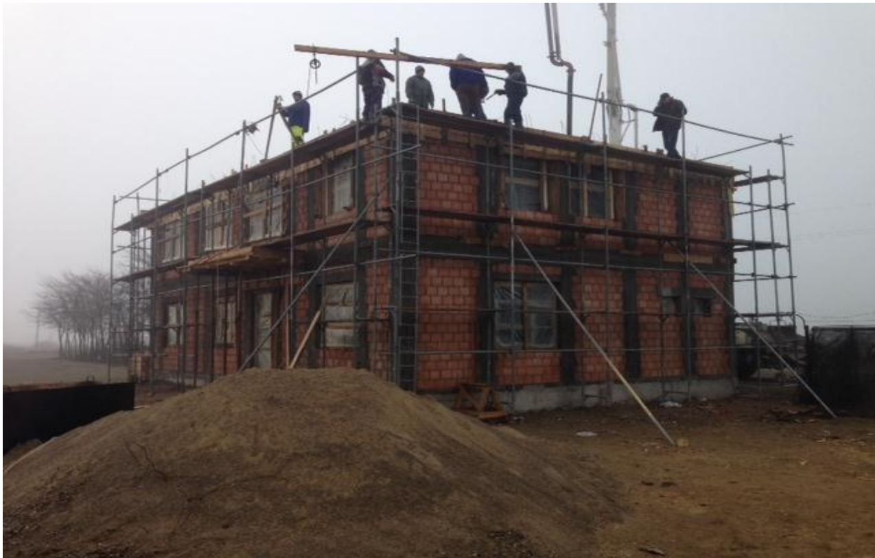
Construction of office building at site in East Romania
