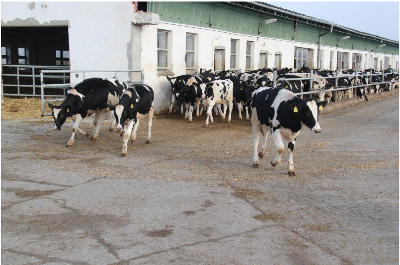
Young cattle stable in Slovakia (under renovation)
